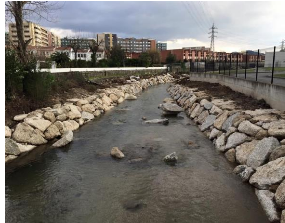
Fig. 12 “Este” River, Focus on riverbank nature-based engineering solutions that increased stability
